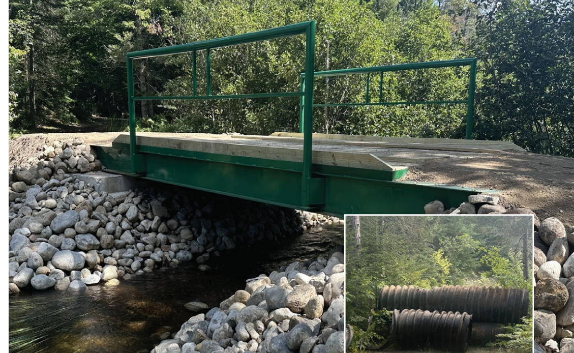
A new clear-span bridge over Casey Creek installed by HRC.; The previously failing culverts at a Fox River crossing that were replaced by clear-span bridges.
